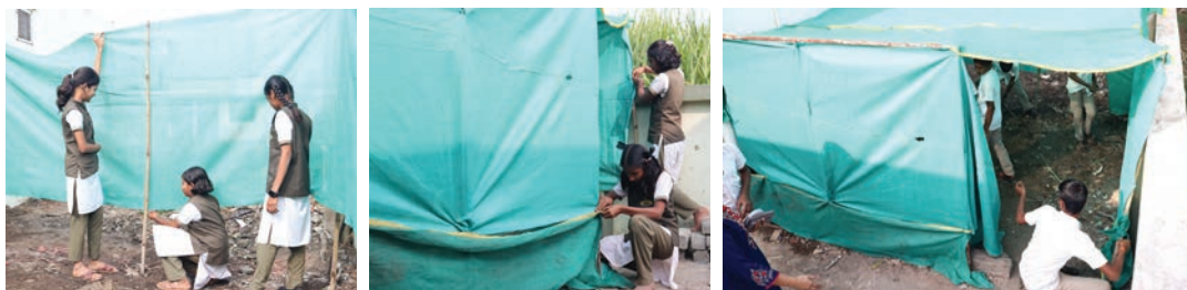
Figure 1.10: Installing the green shade-net
