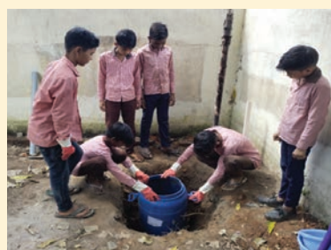
Figure 6.8: Students making a soakpit
